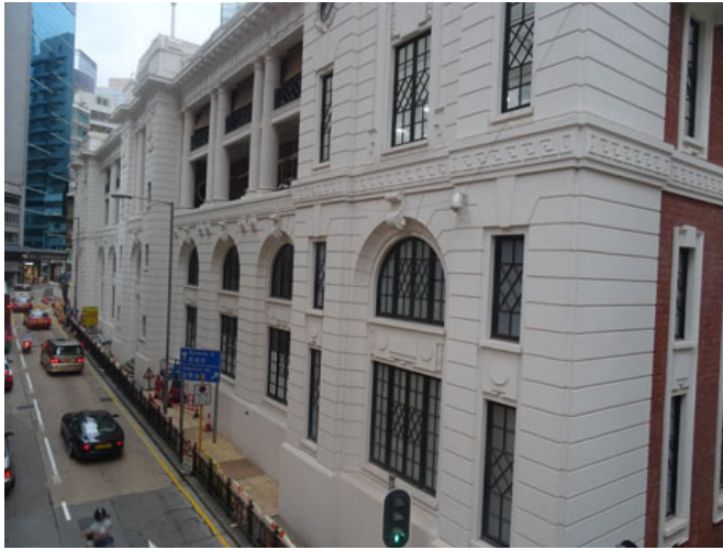
The renovated exterior of the former Central Police Station viewed from the footbridge over Hollywood Road The building is now subject of a conservation and revitalisation project
