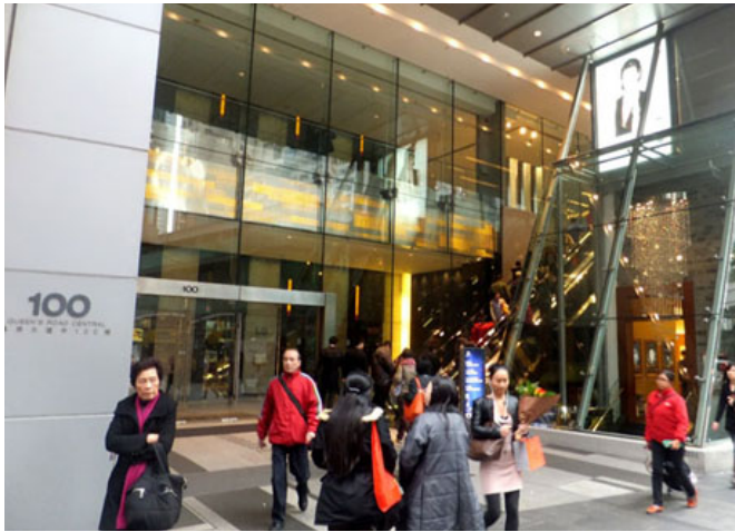
100 Queen's Road, Central. An escalator to immediate right of the main entrance leads to the beginning of the Central - Mid-Levels escalator system
