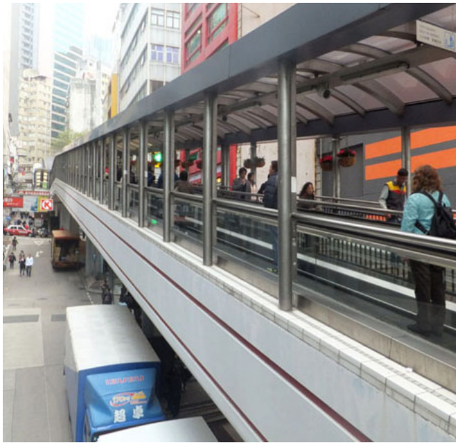
The first section of the system is a moving walkway running up Cochrane Street to Wellington Street
