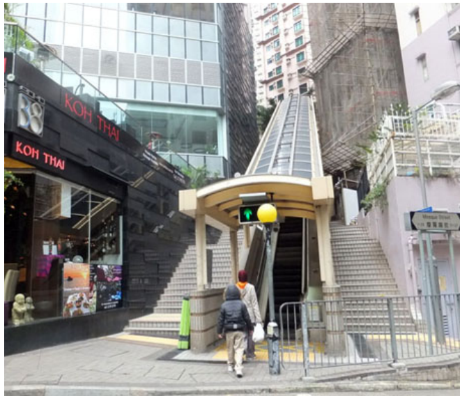
The final series of escalators from Mosque Street to Conduit Road
