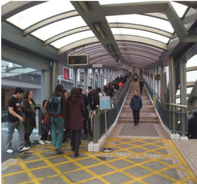
The beginning of the system above 100 Queen's Road Central
