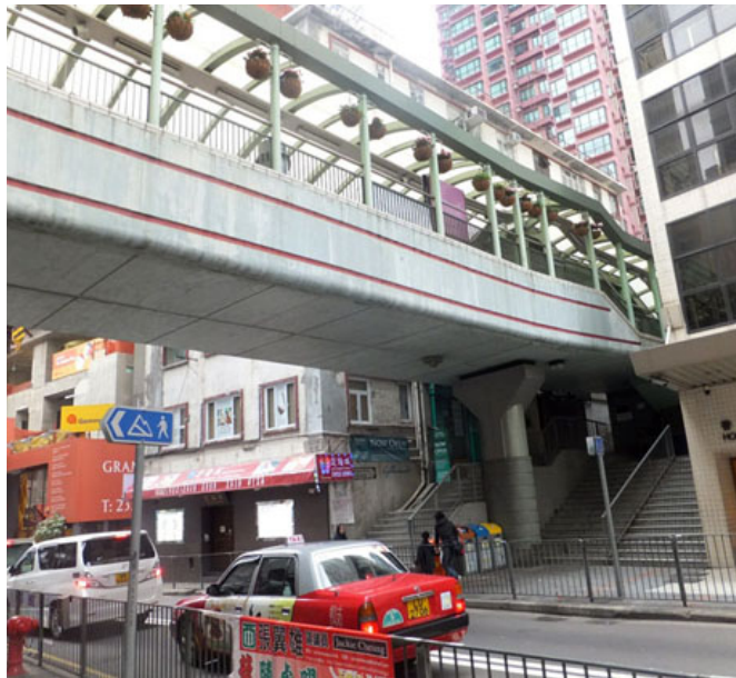
Footbridge over Caine Road, linking the escalators
